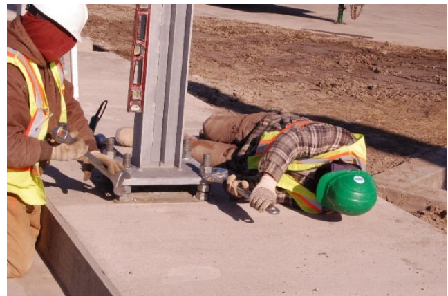
Figure 17 – Tightening of Anchor Rod Nuts
