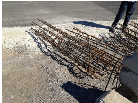
Figure 13 – Assembled Reinforcing Cages
