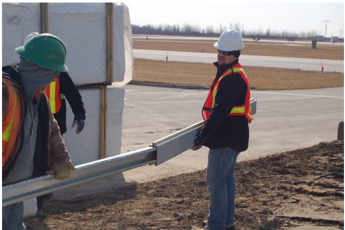
Figure 19 – Inserting C Channel in Bottom Panel
