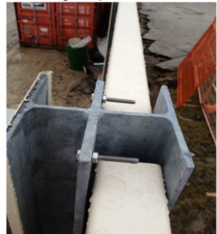
Figure 24: Installed Retention Bolt
