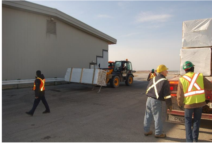
Figure 9 – Forklift Device Handling Panels
