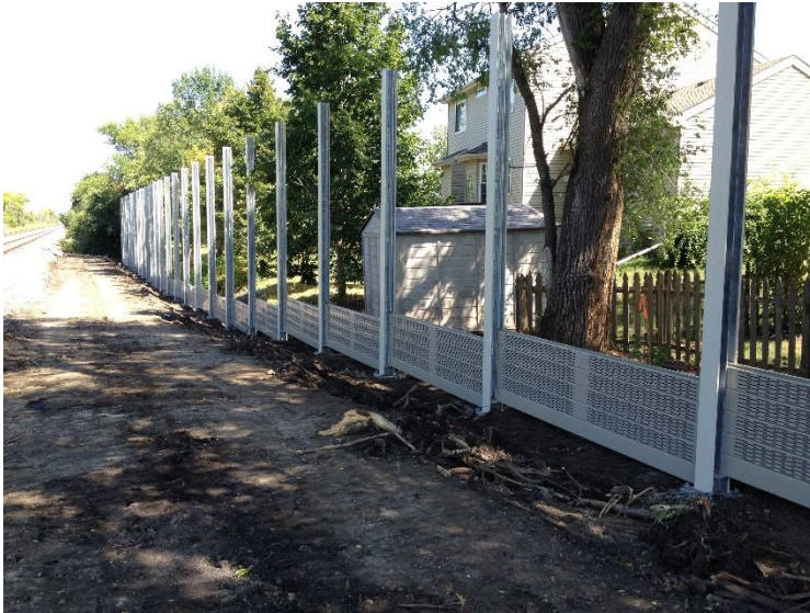
Figure 20 –Panels Installed Near Ground by Hand
