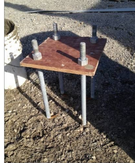
Figure 14 – Anchor Rod Template
